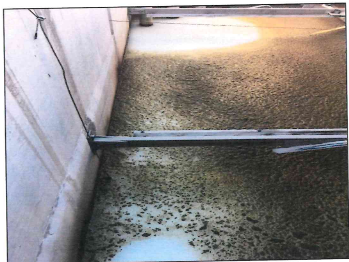
Figure 3. Dissolved Air Flotation Cell (City of Waco)
